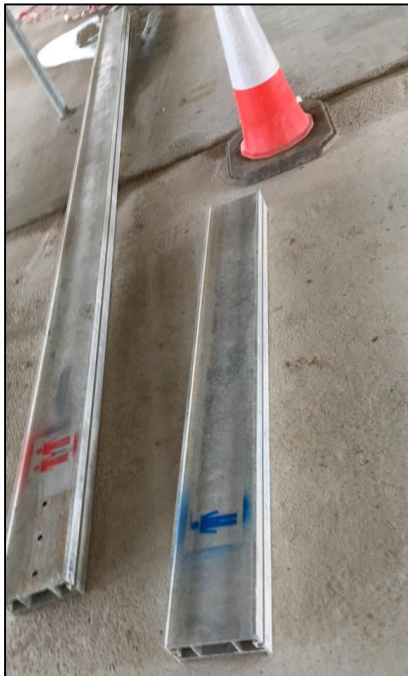
Beams stencilled to indicate individual or team lift
